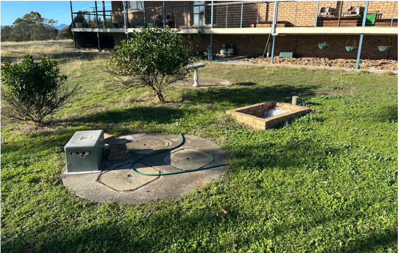
Photo 1: Field photo showing existing Envirocycle on Lot 1.
