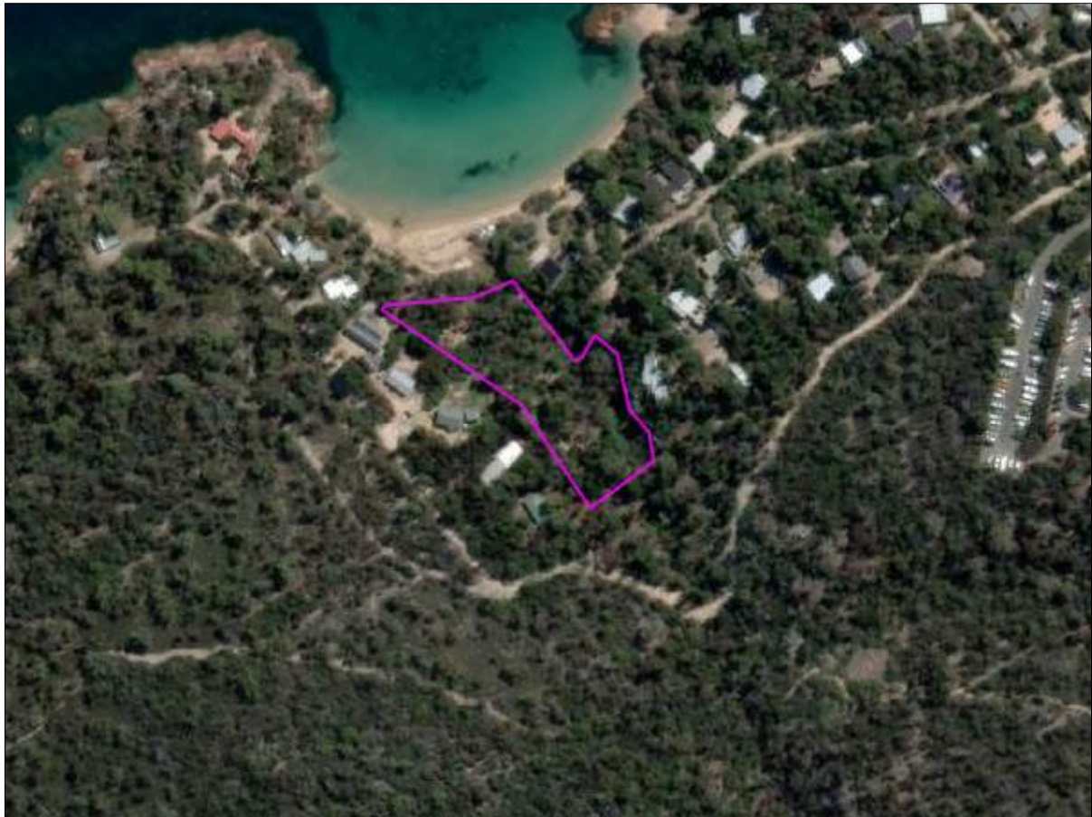
Figure 2. Aerial image of the lot (pink line) showing forest, woodland and low threat vegetation within and adjacent to the lot.
