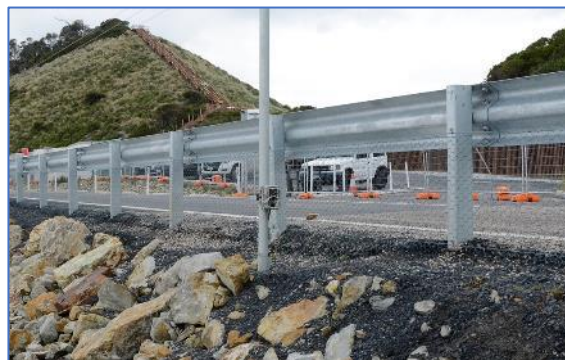
Figure 5: Roadside fencing to prevent Little Penguins accessing the road surface in 2018. A camera trap to record penguin behaviour along the fence line is visible. ©Eric J Woehler.
