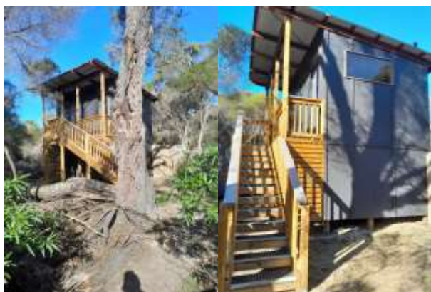
Figure 2 - New toilets at Cooks Beach
