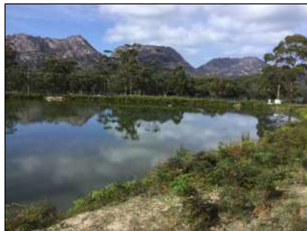
Figure 3 – Existing Freycinet National Park Sewage Treatment Plant
