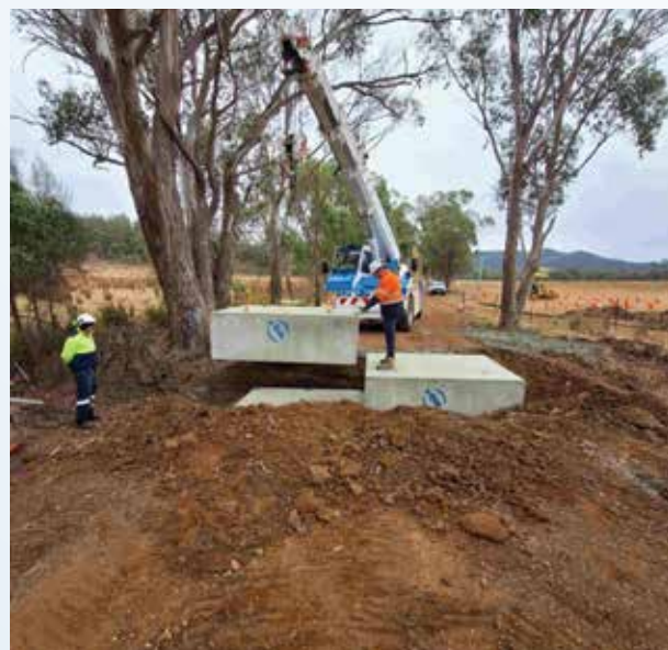
Earlham Road - Stormwater Upgrade
