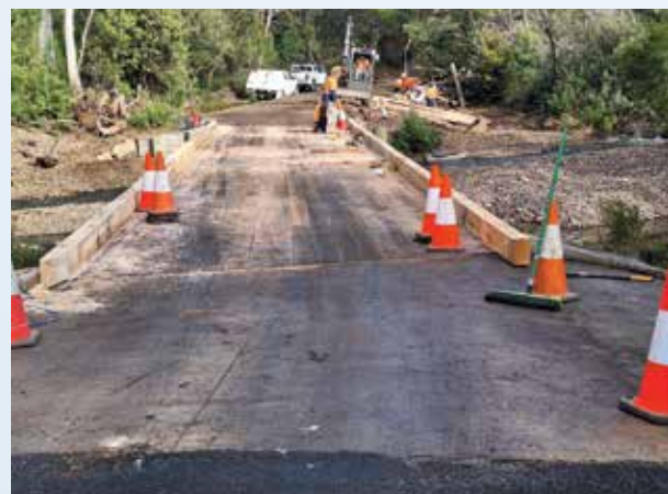
Redecking Rosedale Road Bridge, Bicheno
