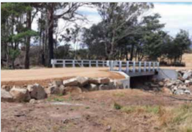
Rheban Road bridge before additional safety barriers installed.
