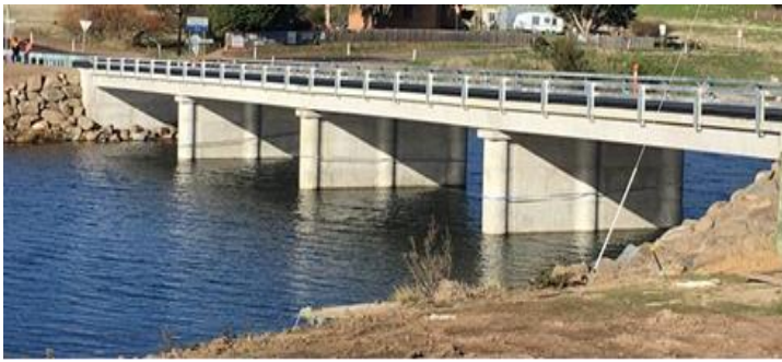
Image of a typical bridge
