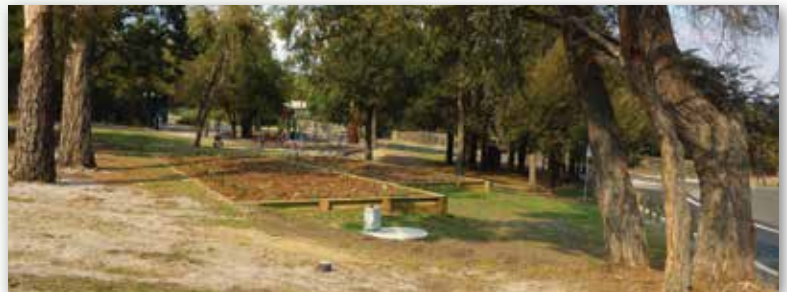
Coles Bay Sub-Surface Irrigation Beds
