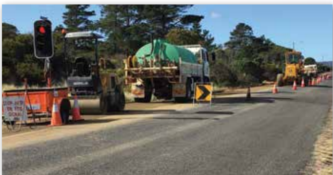
Dolphin Sands Road road widening shared pathway
