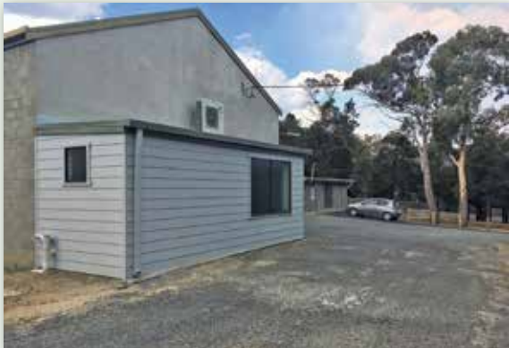
Coles Bay Community Hall Disabled Toilet Extension
