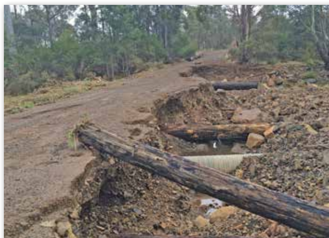
Creek crossing damage - Wielangta Road, Earlham
