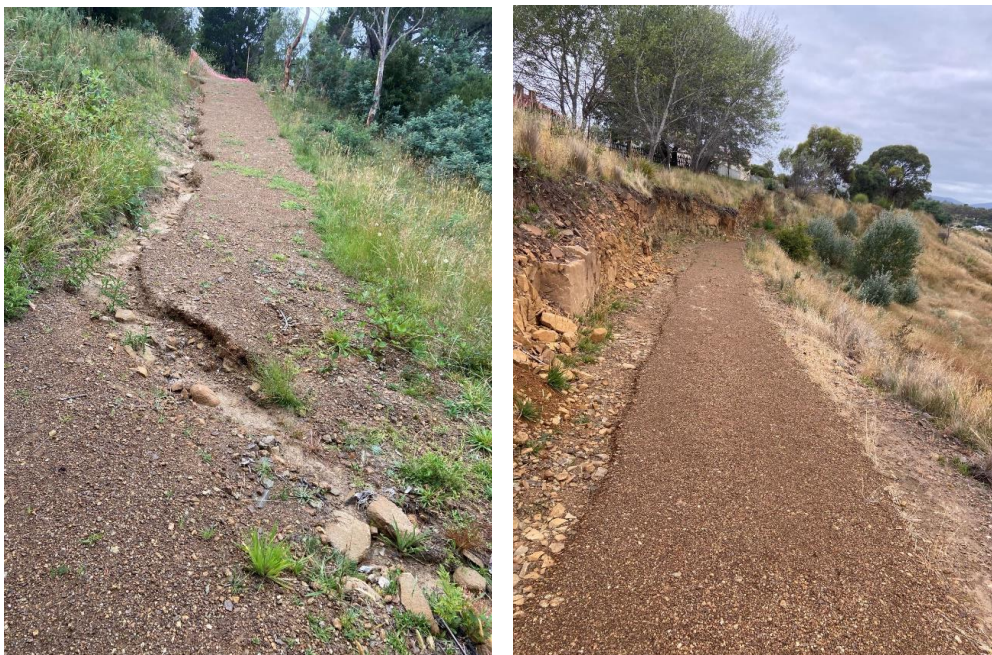
Photo's: Erosion controls required to manage storm water
