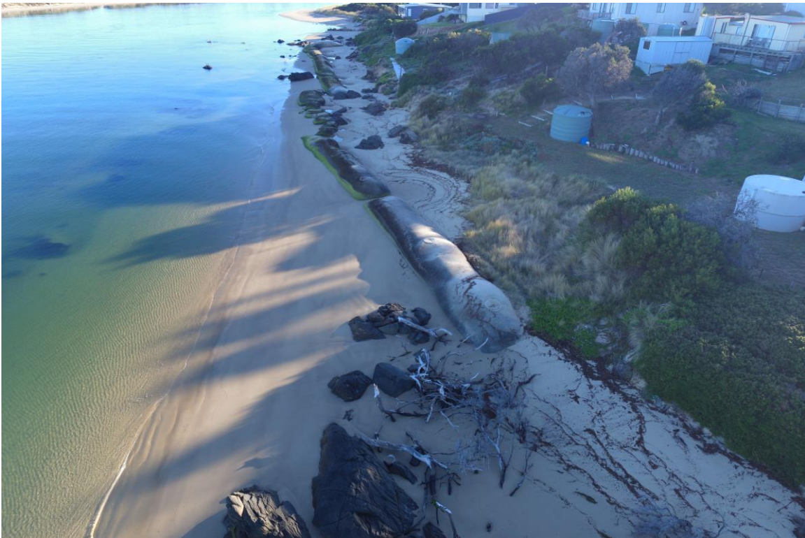
Geo-fabric bags already installed Looking North from 90 Swanwick Drive to Beach access
