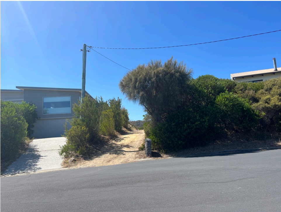
Figure A1-2: Existing shared access from Swanwick drive. Access must be upgraded to comply with bushfire standards before any new dwellings are constructed that are reliant on this access.
