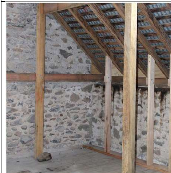
Figure 4: Interior of first floor showing timber roof and flooring construction with stone walls
