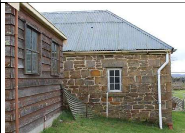
Figure 4: Rear outbuilding of stone construction with hip roof
