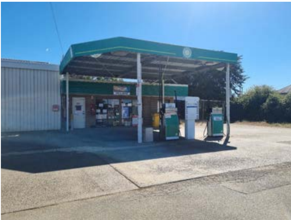
Figure 8. Looking north at the site of the proposed replacement 6 hose dispenser and relocation of the outdoor payment terminal.
