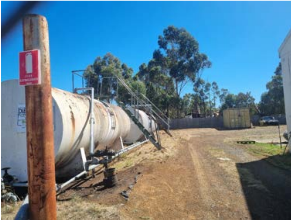
Figure 7. Looking north at the site of the proposed underground fuel storage tanks replacing the existing tanks.
