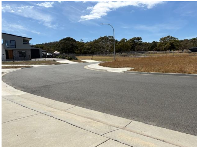
Figure 13– Looking left along Kunzea Circuit from 70 Kunzea Circuit
