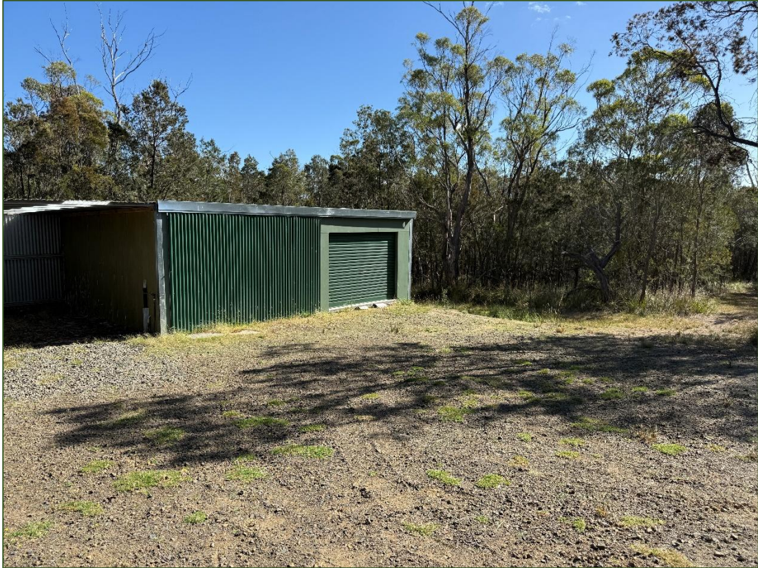
Plate 4. View north of existing shed and associated clearing
