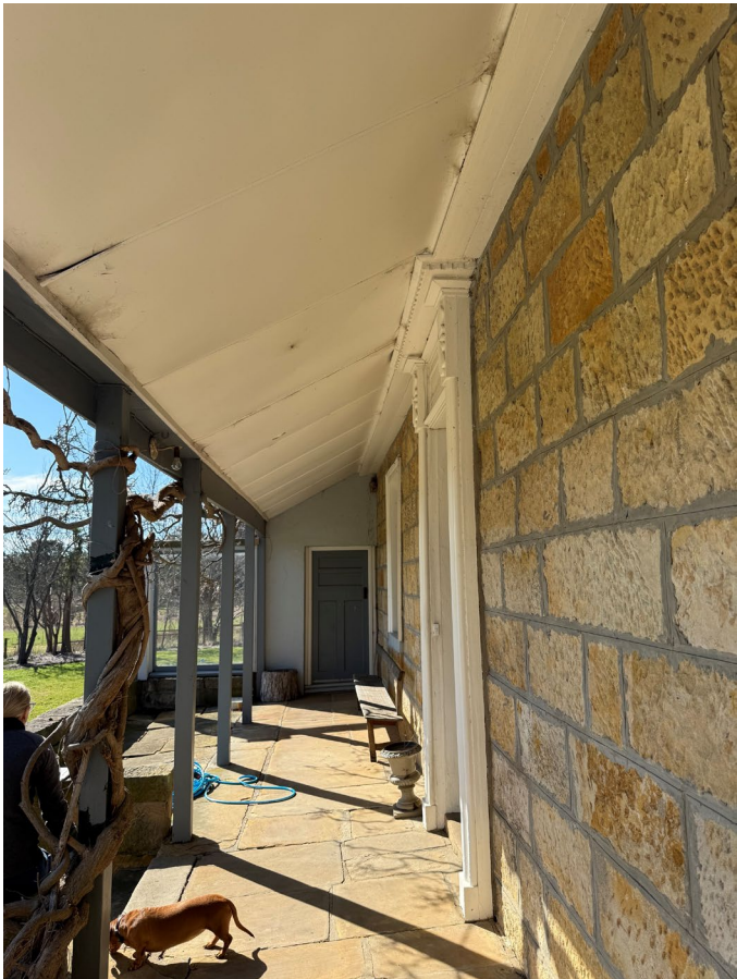
Figure 8: North west verandah appears to be modified from a lined eaves detail to later include a verandah (Source: Taylor + Hinds)
