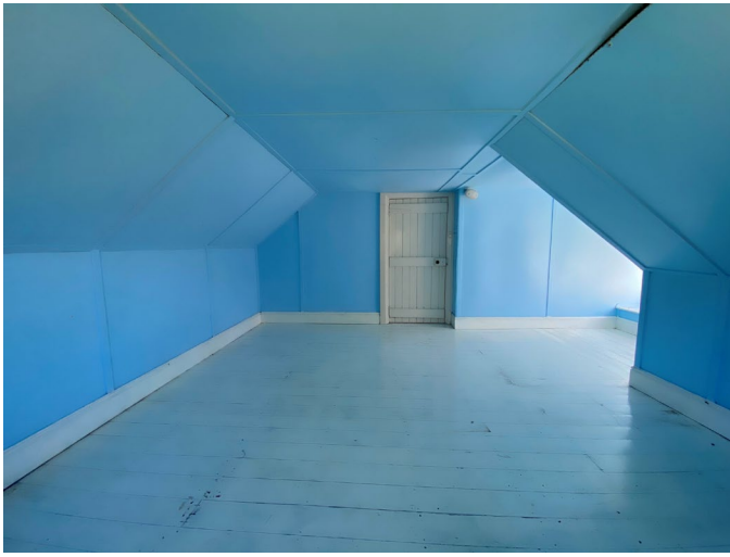
Figure 11: Non-original linings to attic nominated for removal. Floor linings nominated for removal and creation of double height rooms (Source: Taylor + Hinds)
