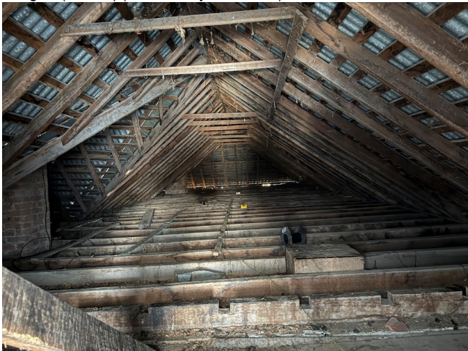
Figure 9: Roof interior of original built form. Notched roof beams to the foreground of the image are assumed to be from previous rafters, corresponding with the far end hip (Source: Taylor + Hinds)
