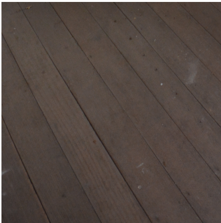
E.FB1 EXISTING FLOORBOARDS. SELECTIVE REPAIR AS REQUIRED. WAX FINISH TO FUTURE SPECIFICATION
