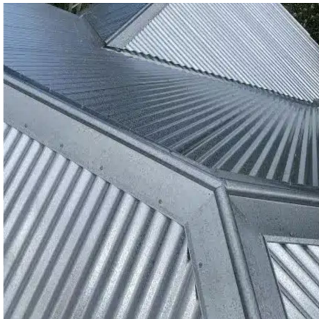
RS1 HERITAGE GALVANISED Z600 SHEET ROOFING. 20mm BARRELL ROLLED PROFILE
