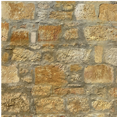
E.ST1 EXISTING SANDSTONE WALL. SELECTIVE REPAIR AS REQUIRED.
