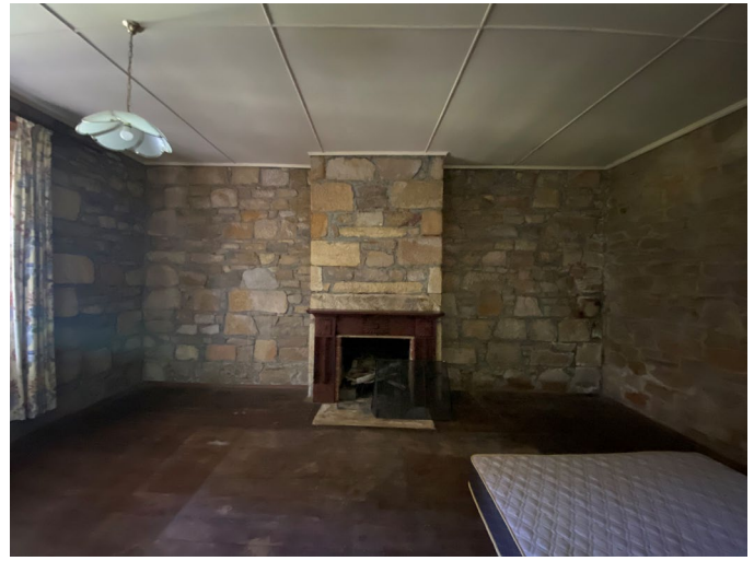
Figure 12: School room with exposed stone walls and cement pointing. (Source: Taylor + Hinds)
