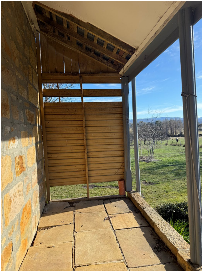
Figure 7: North east verandah with outrigger rafters and closely spaced battens. Presumed to have been previously finished with timber shingles (shakes) (Source: Taylor + Hinds)
