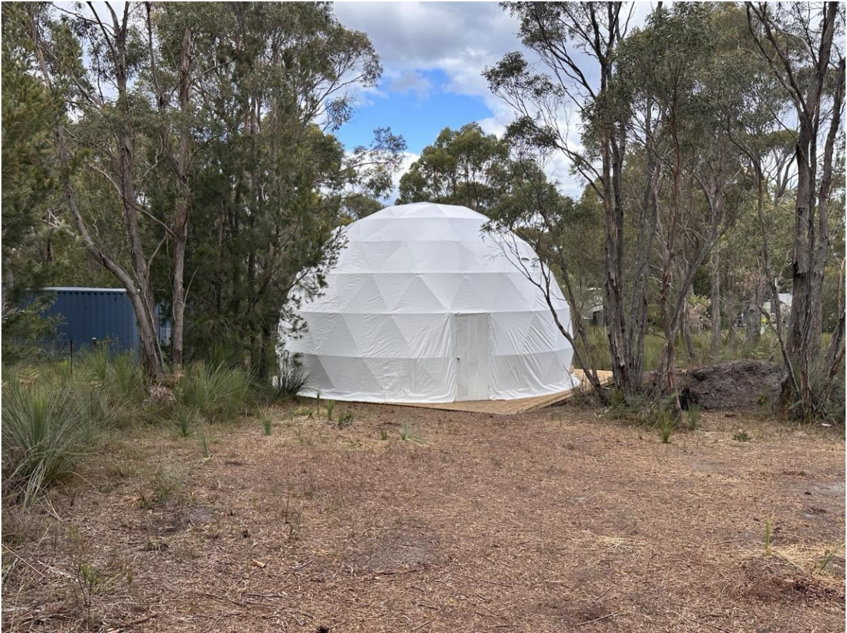
3 x geodesic domes on timber decks for private camping 1 Happy Valley Rd, Spring Beach
