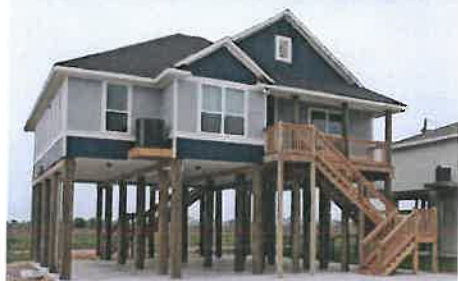
Raising houses for flood protection
