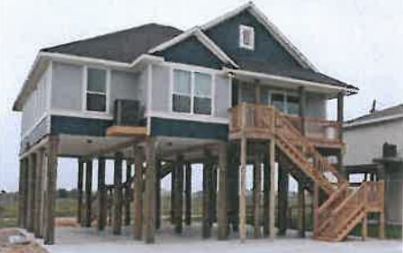
Raising houses for flood protection
