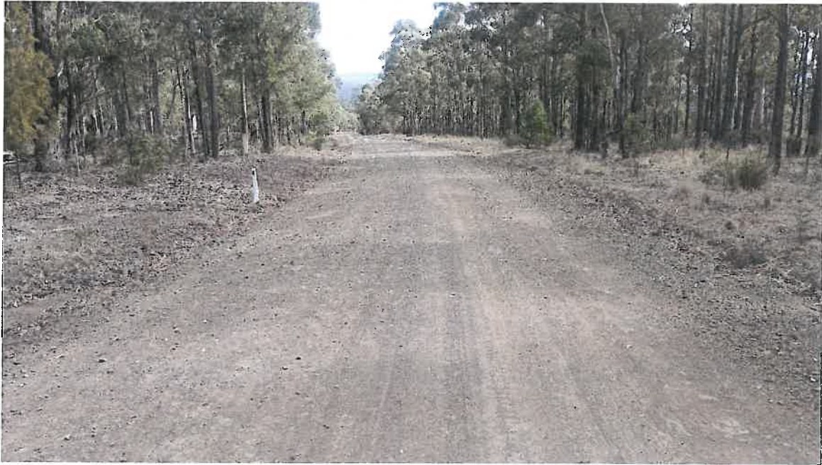
Figure 5 – Roadside drains and vegetation rated as Low level demand
