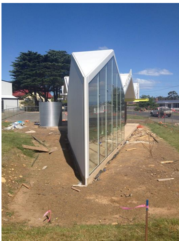
Image: Triabunna Gatehouse under construction
