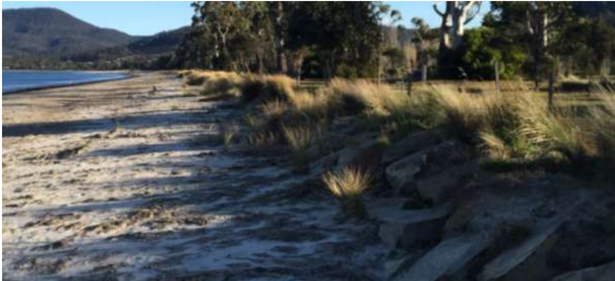
Figure 17 Rock revetment at Raspins Beach, Orford
